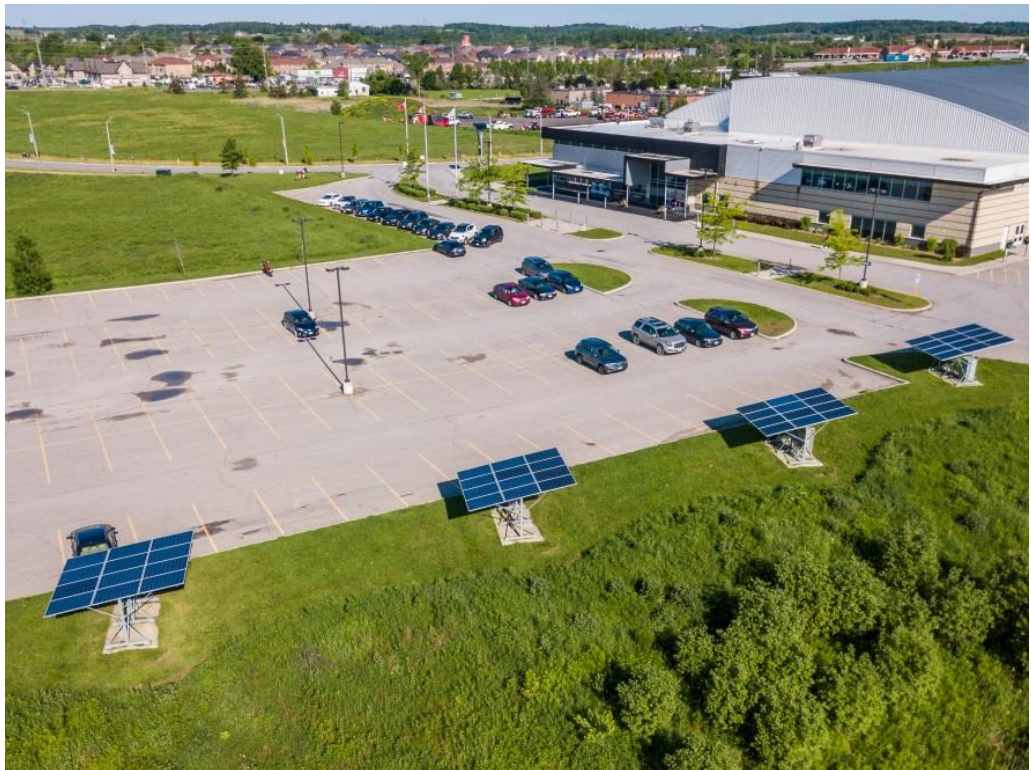
Solar MICROFIT array at Trisan Centre Photo taken by HAV Photography
